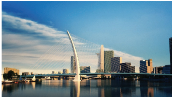
Thu Thiem 4 Bridge
