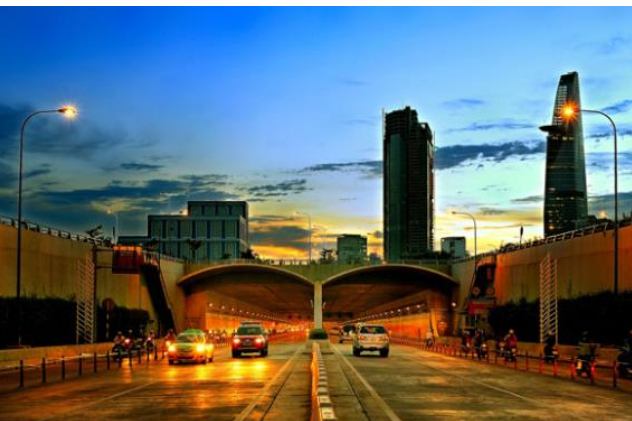
Thu Thiem Tunnel
