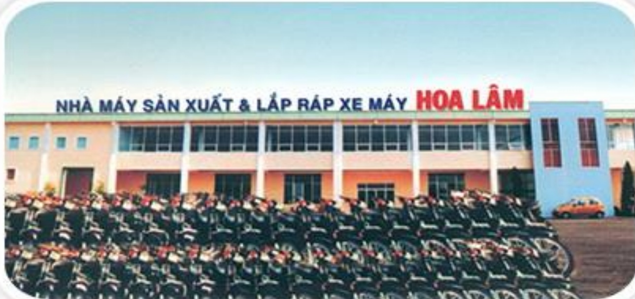
Hoa Lam Manufacturing and Assembly Factory
